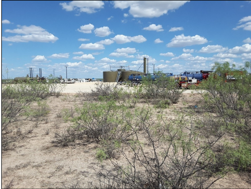
Figure 6. Medallion facility at the southern terminus of the project area, view south.
