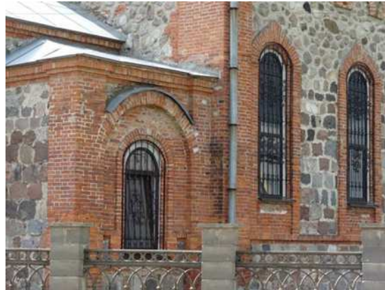
Fig. 1. Fragment of masonry
