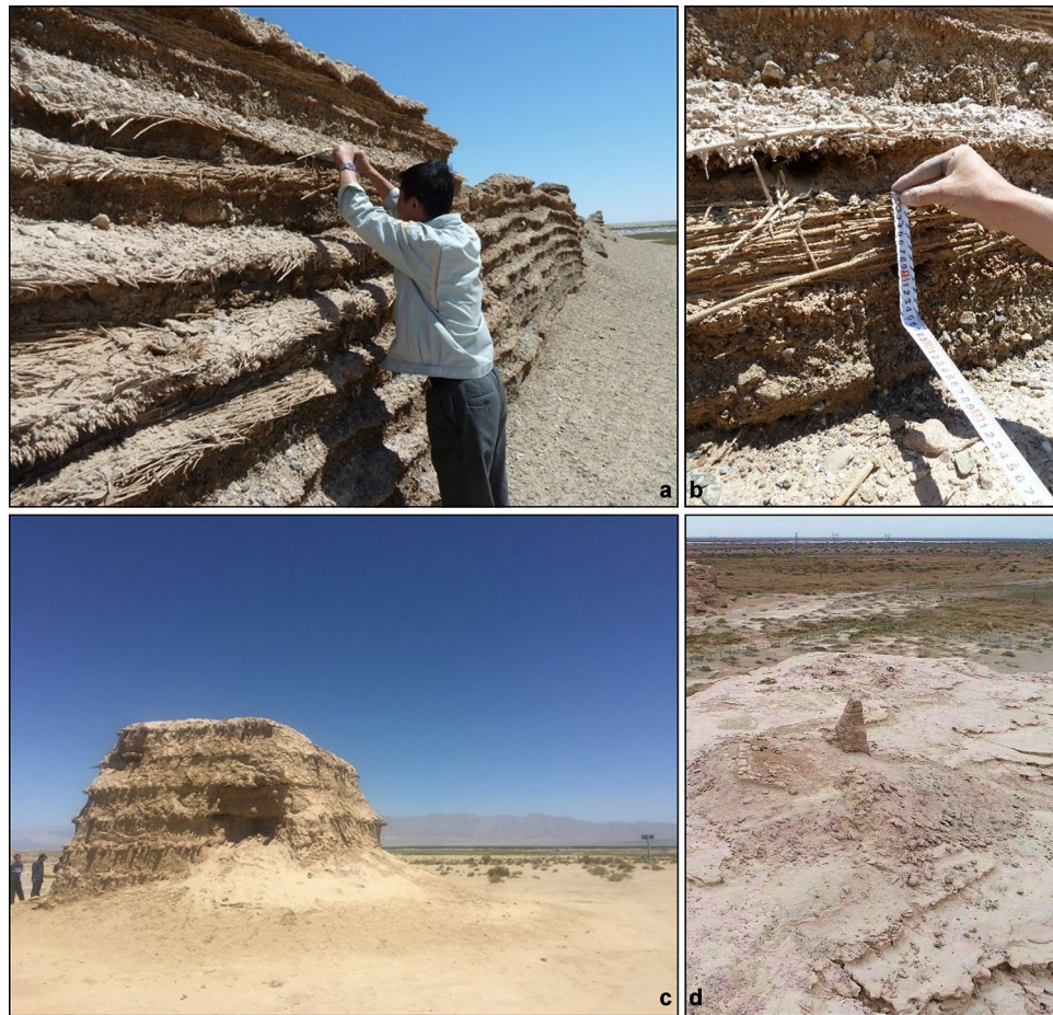
Figure 2. Remnant wall segments and beacon towers of northwestern China. (a) Sampling of Phragmites culms from a wall section at Majuanwan (Site 7); (b) Reed fascines alternating with layers of rammed earth at Majuanwan. Near center is a fascine of Phragmites culms that were sampled for analysis; (c) Remnants of Sishilidadun Beacon Tower (Site 14) dating to the Song Dynasty. Although not visible, the beacon tower was constructed like the wall section in panel a, with rammed earth alternating with reed fascines; (d) Low altitude air photo of the Yakelun Beacon Tower (Site 11), courtesy of Xingjun Hu. Note the wild plants growing adjacent to the tower.
