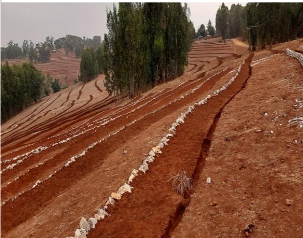
Stone faced graded soil bund in Wogera woreda, Amhara region, photo credit by Enideg Dires
