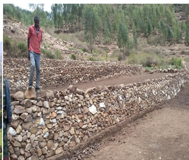
Stone bench terrace at Haramaya woreda (Oromia region), photo credit by Yatu Chalesa
