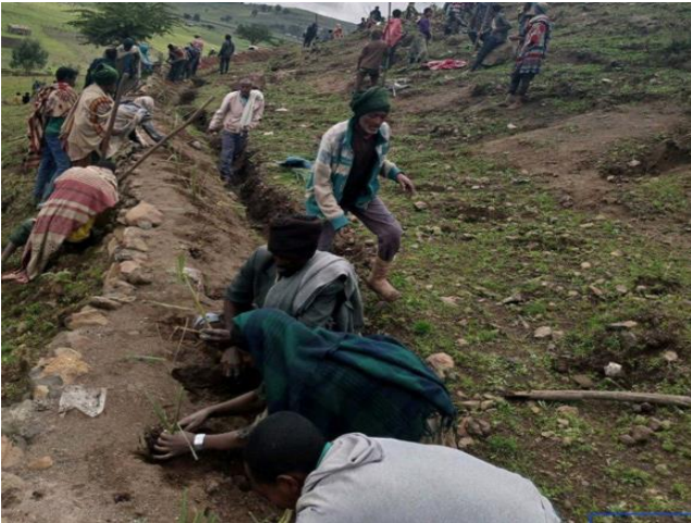
Stone faced graded soil bund in Wogera woreda, Amhara region, photo credit by Enideg Dires
