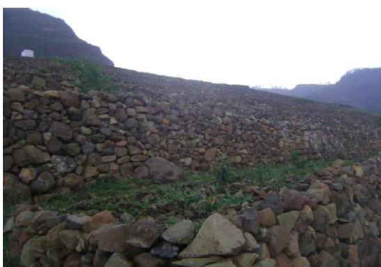
Stone wall bench terrace in Endamehoni (Tigray region), photo credit by Zenebe Adimassu
