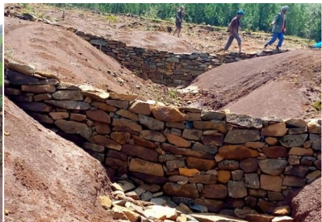
Loose rock check-dam in Amhara Region, photo credit by Shibabaw Goshu
