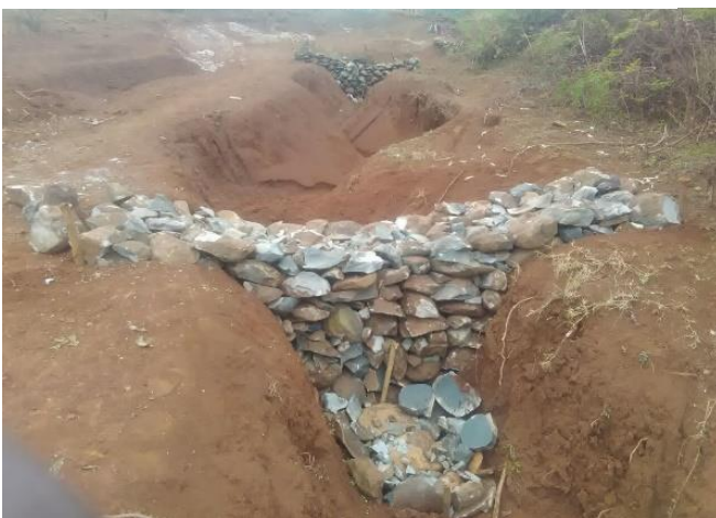
Loose rock checkdam in Oromia region, Kelem Wolega by Mubarek Ahmed
