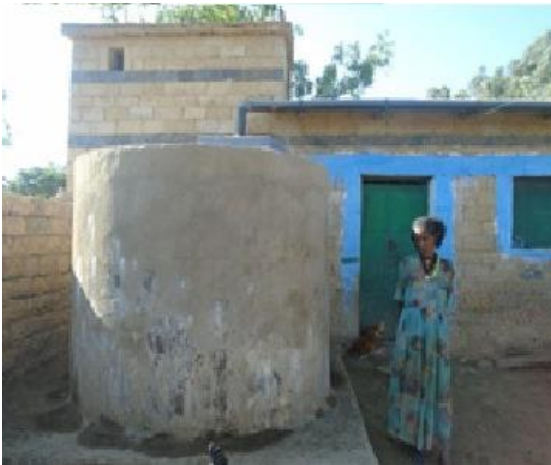
Roof water harvesting in Tigray at Kolla Temben by Mulu Haftu
