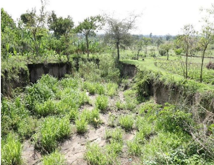
Gully rehabilitation using live checkdam in Hawassa Zuria woreda (Sidama region), photo credit by Esayas
