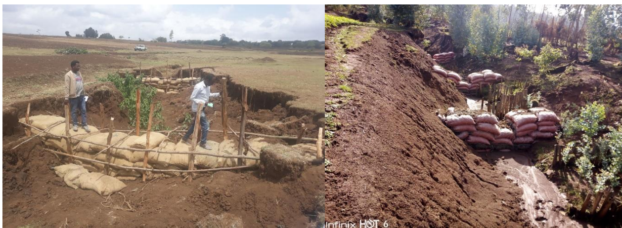
Sandbag checkdam in Takusa woreda, Amhara region, photo credit by Angaw Zewdu
