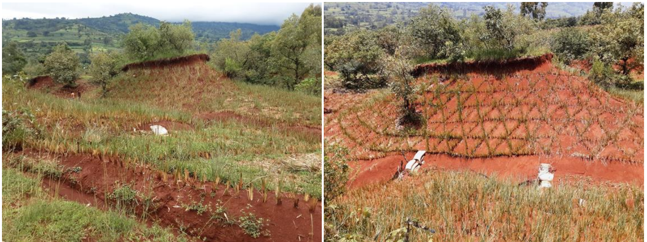
Gully wall reshaping and revegetation in Jimma ( Oromia region), photo credit by Leta Hayilu
