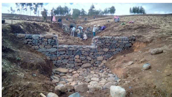
Checkdam in Debark woreda, Amhara region, photo credit by Alemu Birhanie
