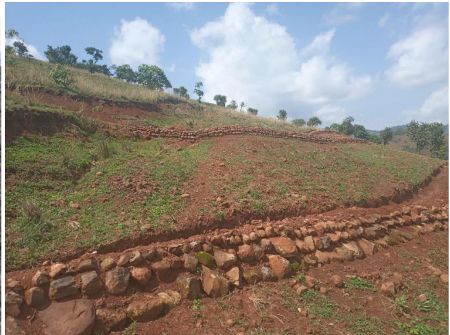
Stone-faced level soil bund in Oromia region, Wara Jarso woreda by Bonsa Lemi
