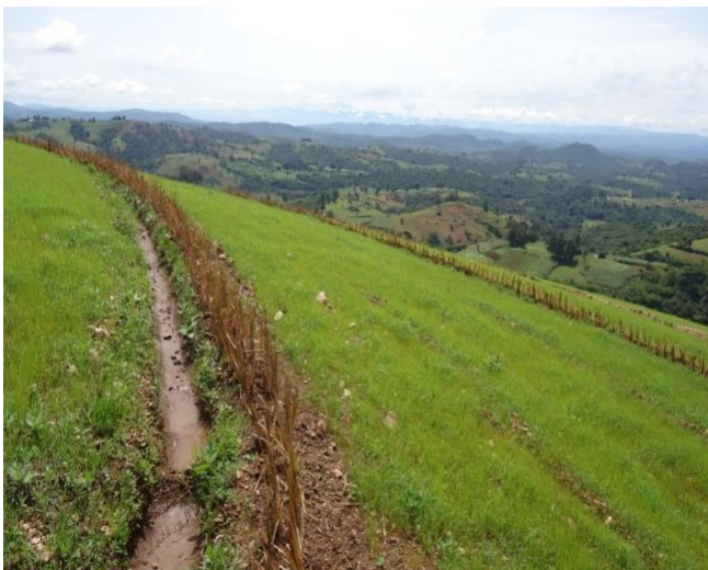
Graded soil bund with Vetivar grass at Haru woreda, Oromiya region, photo credit by Leta Hailu
