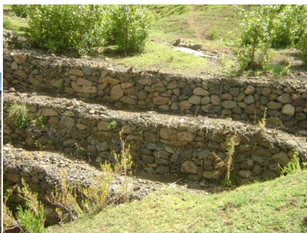
Gully head treatment using gabion in Endamehoni woreda, Tigray region, photo credit by Zenebe Adimassu
