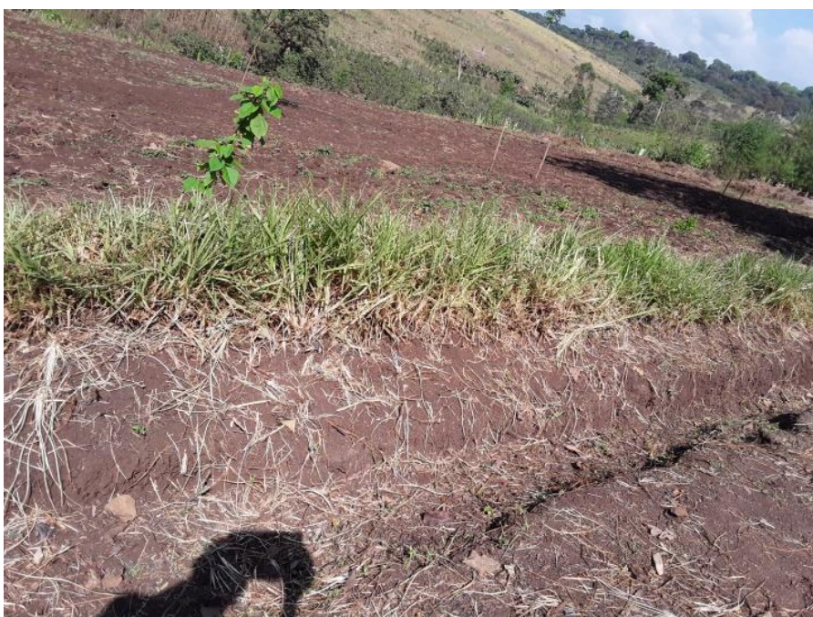
Cut-off drain in Mengesh woreda (Gambella region), photo credit by Mikre Adane
