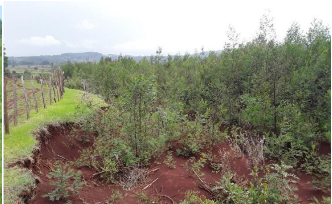
Gully stabilization using vegetation in Bure Zuria Wereda, Amhara region, photo credit by Melsew
