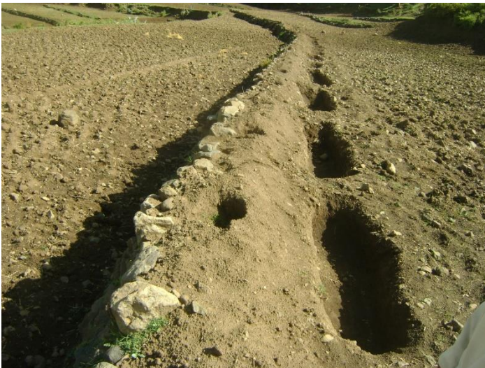
Stone-face level soil bund with trench in in Endamehoni (Tigray region), photo credit by Zenebe Adimassu
