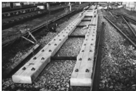
(e) ladder sleepers (Miura et al., 1998)
