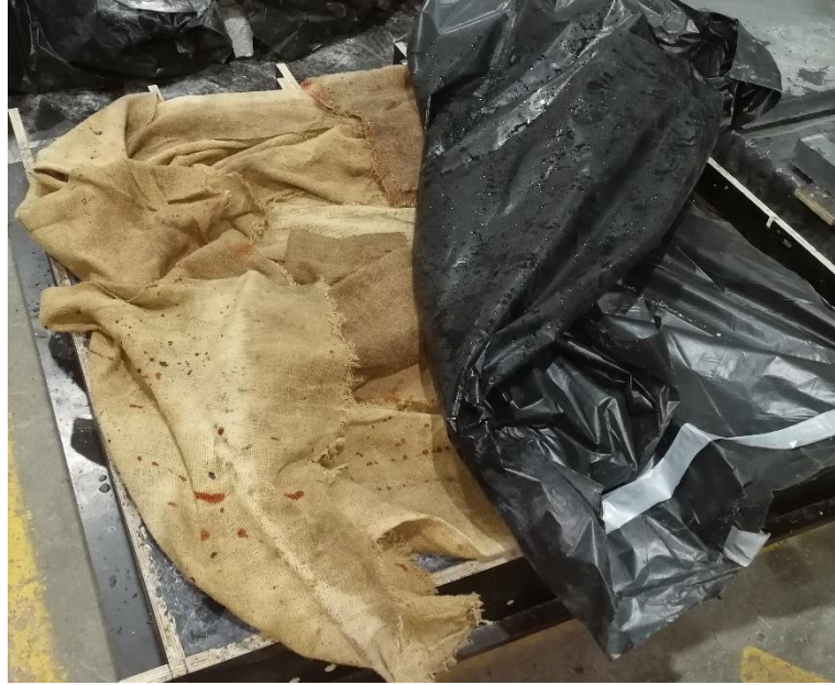
Figure 6.4 Covering the UHP-FRC prototype sleepers with wet hessian and plastic sheets
