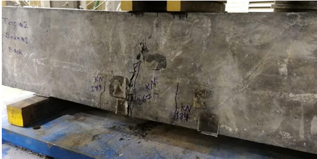
(a) failure mode of S2-S2
