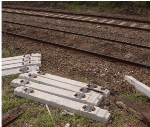
(c) low-profile concrete sleeper (Gallery, 2010)
