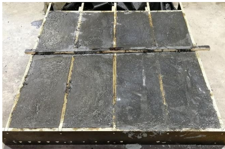
Figure 6.3 The low-height UHP-FRC sleepers, 24 hours after pouring
