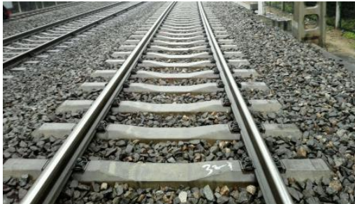
(a) mono-block PSC sleepers (You et al., 2017)
