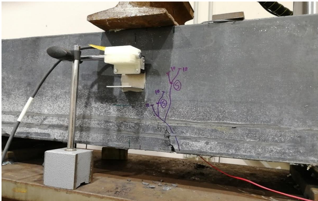
Figure 4.20 The cracking pattern of sample S1-F1 after 10 Cycles
