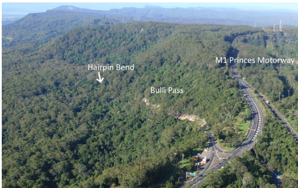
Figure 2: Oblique March 2009 aerial view of Bulli Pass section of the Illawarra Escarpment looking south. The hairpin bend is just left of centre
