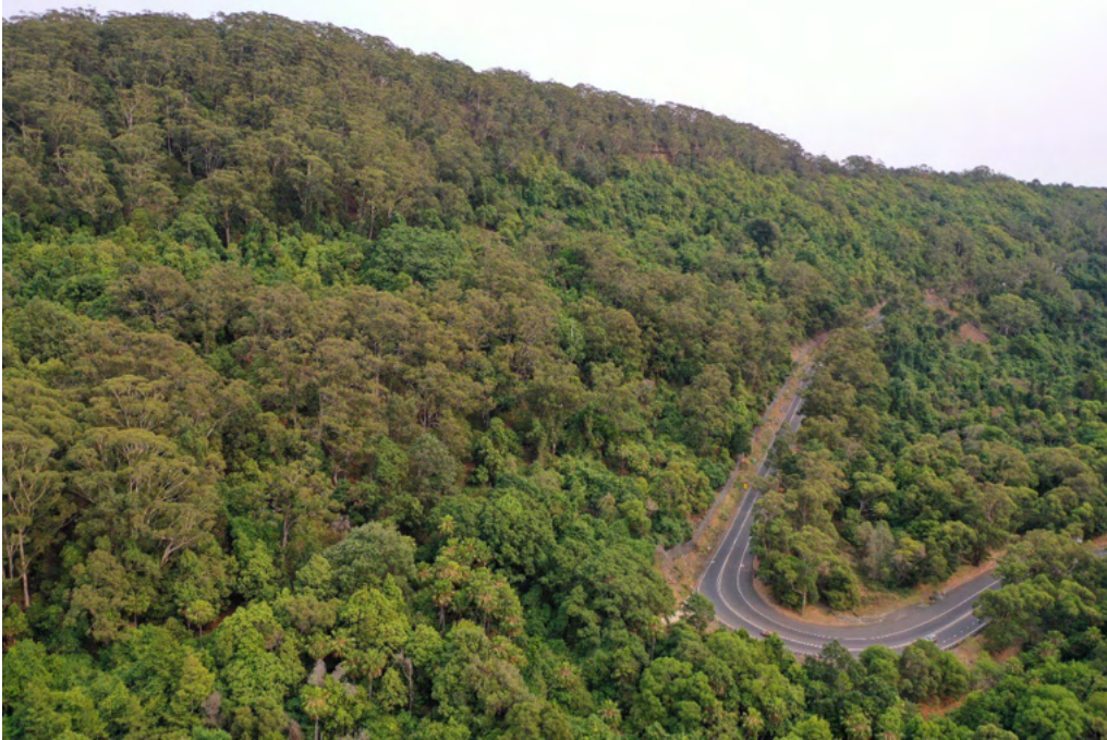
Figure 4: Oblique drone view from south of the hairpin looking north up the pass road and the subject forested slopes above
