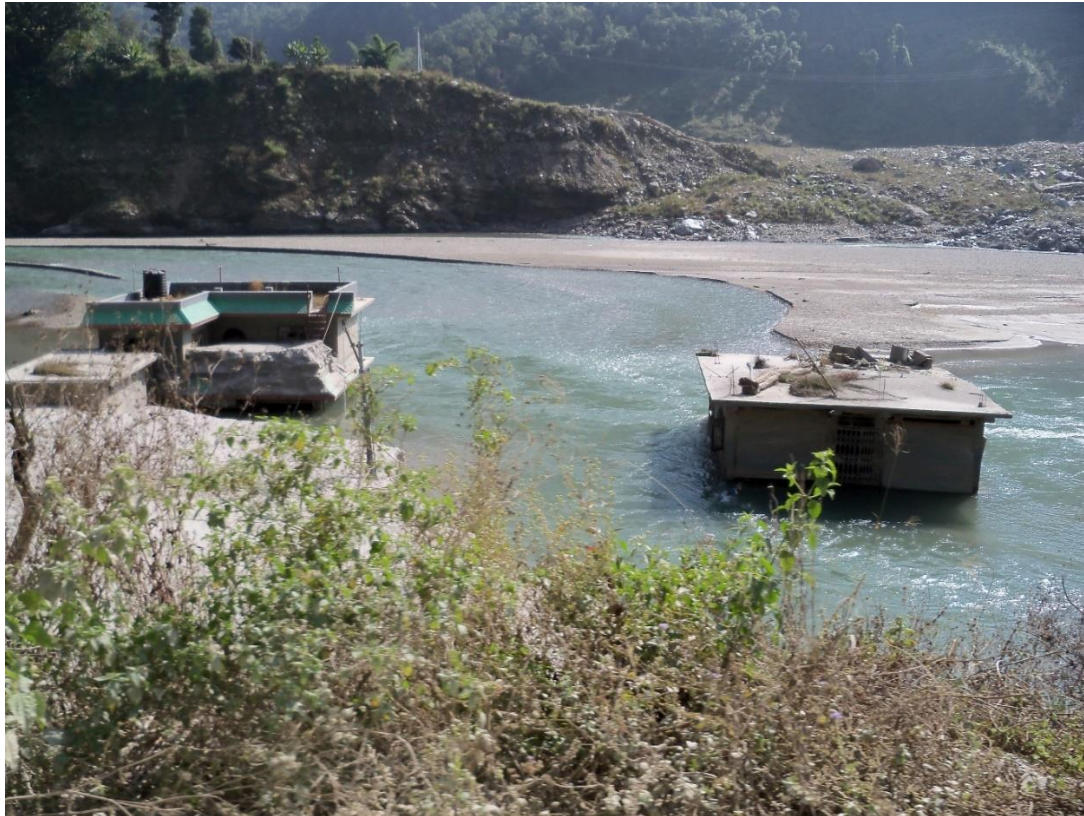
Figure 9- Flooded homes immediately upstream of the 2014 Jure landslide dam in Nepal following the controlled breach and draining of the resulting lake. Sediment deposits on top of the houses shows they were completely submerged by the upstream flooding from the blockage.
