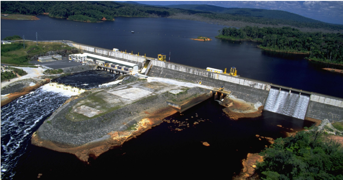
Figure 2: Overview of Petit-Saut Dam (1 July 1995).
