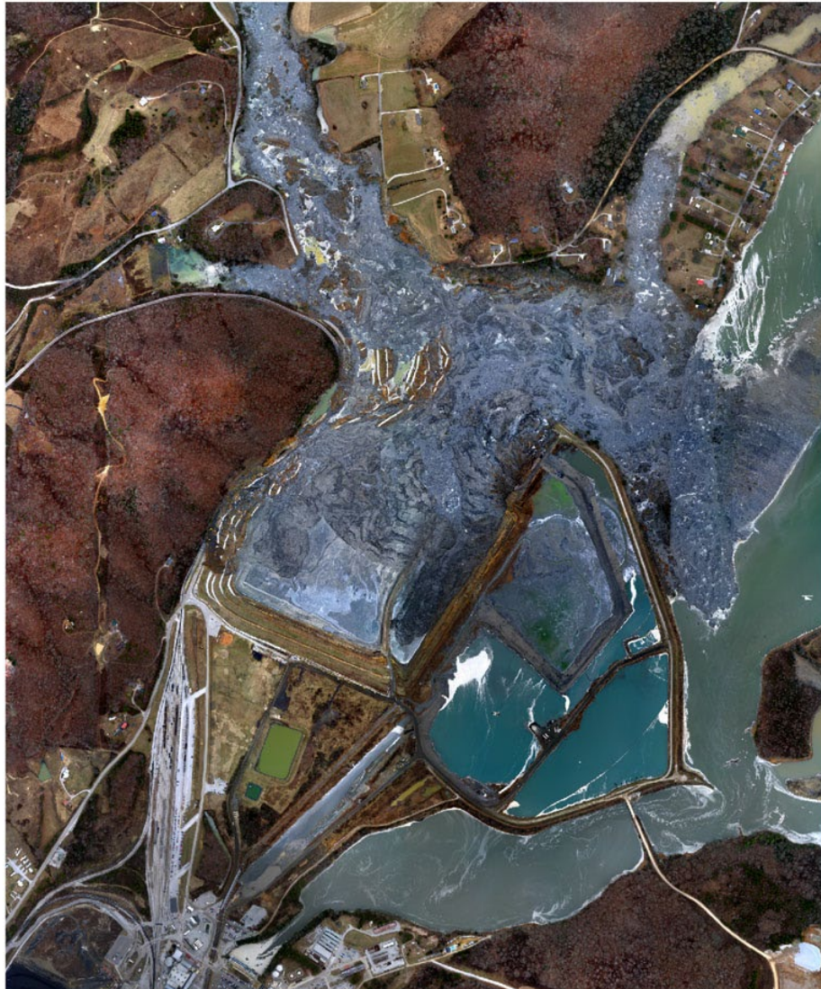
Aerial Image Of Kingston Ash Slide 12/23/08
