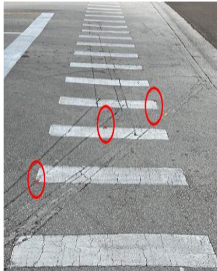
Figure 7 Landmarks on the crosswalk
