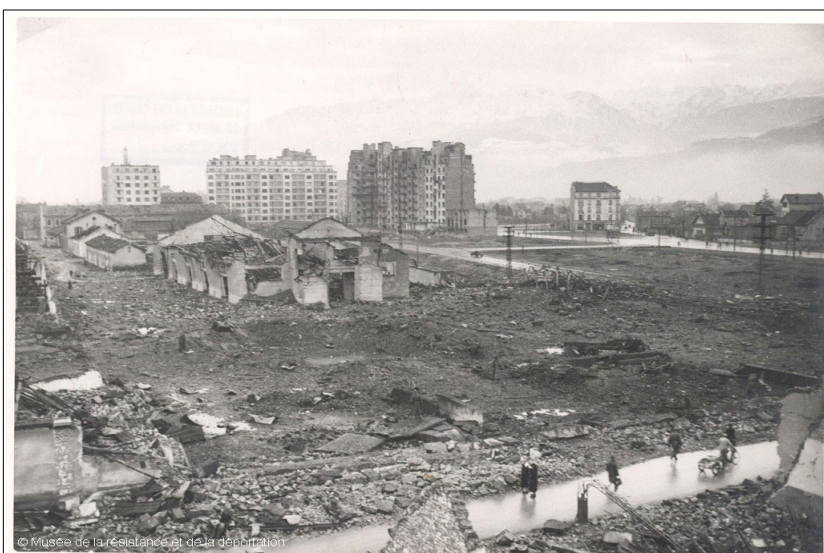
Bonne barracks after the explosion
