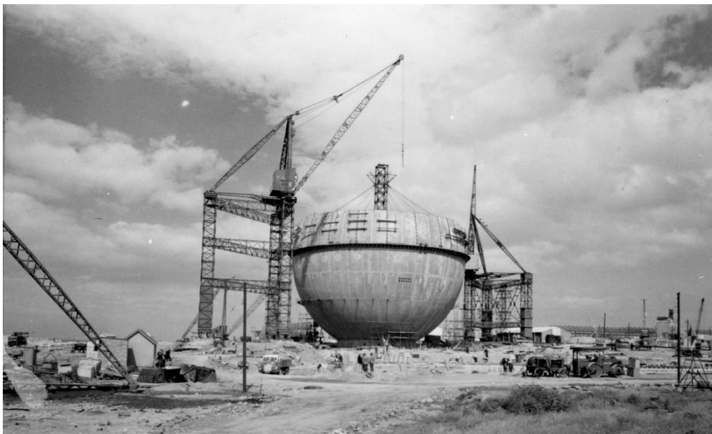
Fig. 2.3: Dounreay Sphere under construction ©Nuclear Decommissioning Authority.
