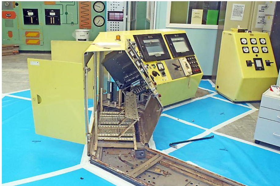
Fig. 2.7: DFR Control Room desk being dismantled in 2013, DFR Condition Report.
