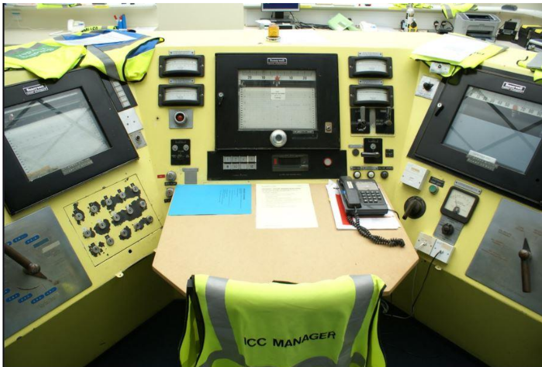
Fig. 2.8: DFR control desk showing wear and adaptations by workers. ©Gair Dunlop
