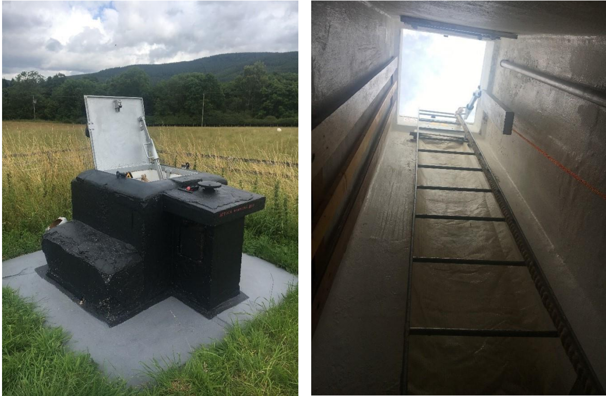
Fig. 3.8: View of the Traquair ROC post hatch and view looking up the ladder. ©Sarah Harper.
