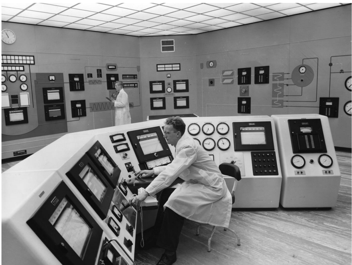
Fig. 2.2: Dounreay Fast Reactor Control Room in operation ©Nuclear Decommissioning Authority.
