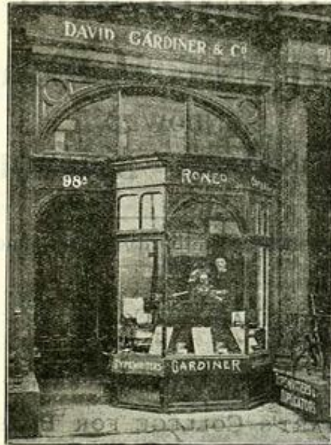
FRONT VIEW OF SHOWROOMS.
