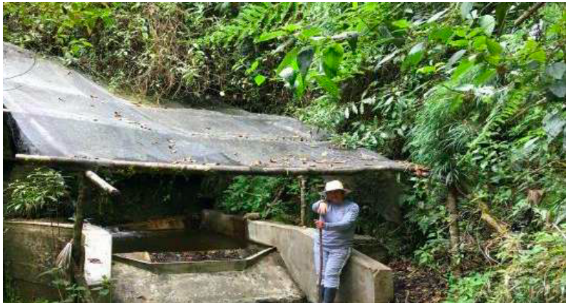
Figure 1: Community aqueduct in Pasto, Colombia (Perugache Salas, 2020).
