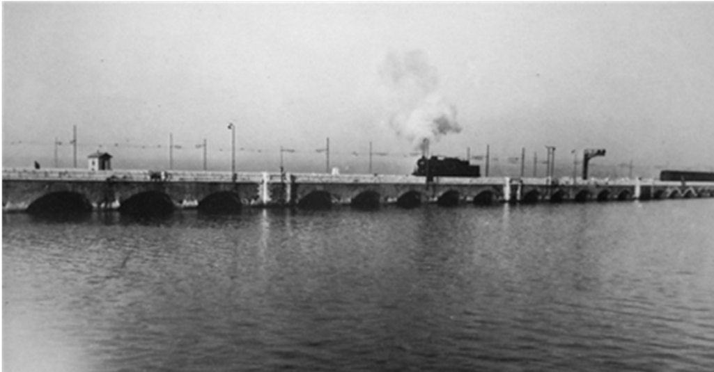
Figure 1: The Venice trans-Lagoon Bridge, Italy, during the XIX century.
