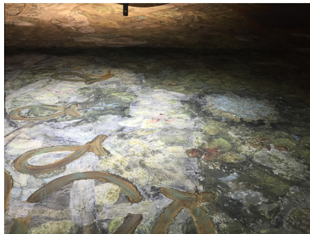
Fig. 4. Polychrome vault: white efflorescences are unevenly distributed forming a whitish covering layer.
