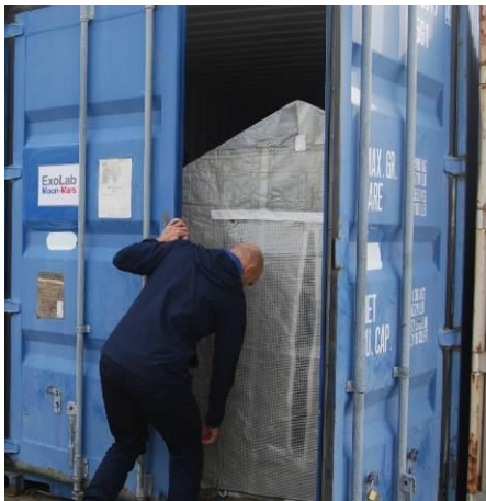
Fig. 7 Airlock to access the ISO container
