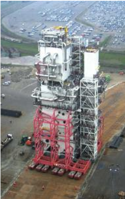
Figure 1.12 - A modularised cold box for an LNG plant at Hammerfest, Norway . The unit, that had a weight of 2700 tons and was 60 meters high, was transported from Belgium to Norway by barge and then a semi-submersible ship. (Source: Fagioli)
