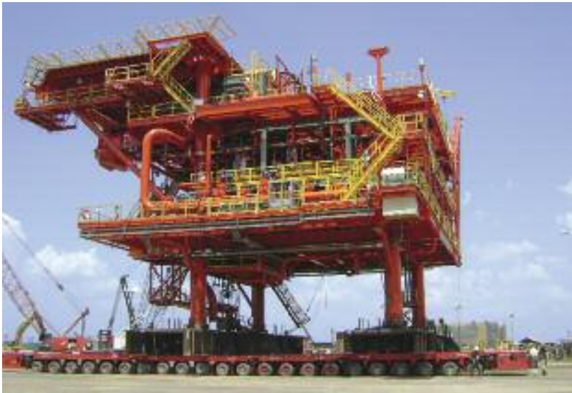
Figure 2.3 - The 25 meters deck of an offshore plant on a Self-Propelled Modular Trailer. (Source: Fagioli)
