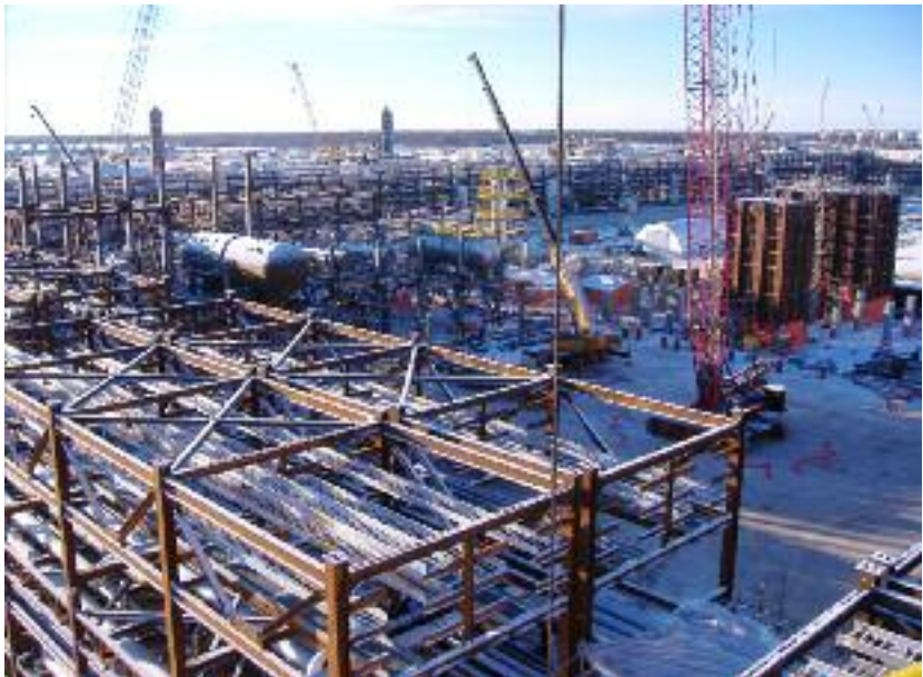
Figure 1.6 - A view of the Horizon Oil Sands Plant, Fort Mc Murray, Northern Alberta, Canada. In the last decades modularisation has been largely adopted in order to mitigate the impact of severe weather conditions at site. (Source: Technip)
