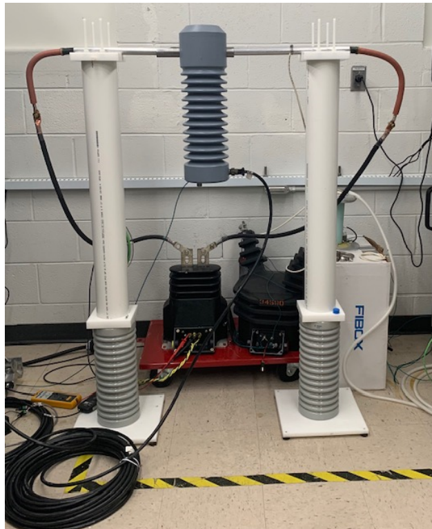
Figure 4.2: Laboratory setup with Lindsey sensor connected to driving CT
