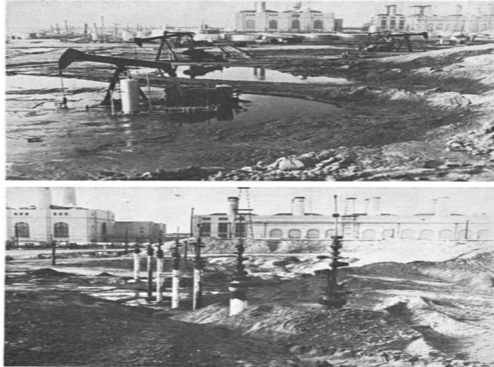
Figure 10: Remedial work near the Long Beach, CA area, (Pierce, 1970).
