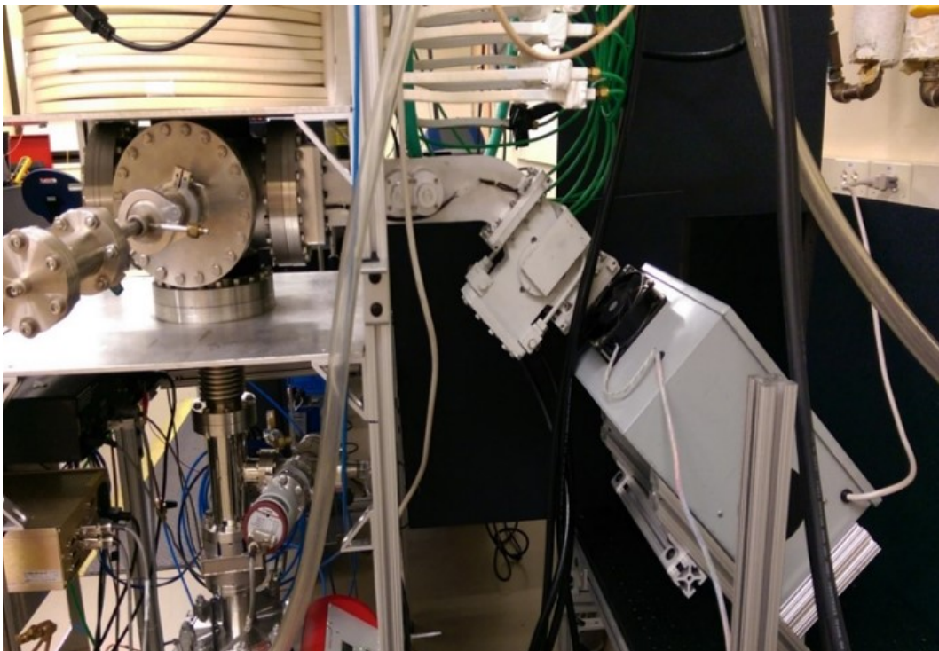
FIGURE 2.10: Photo of the microwave injection apparatus on CHEWIE. The large gray box to the far right is a RF shielded and grounded box that isolated microwave emission from the rest of the laboratory. The magnetron is inside the shielding box. Attached to the box is the circulator with the water-cooled dummy load. Following the circulator is the two-stub waveguide tuner.
