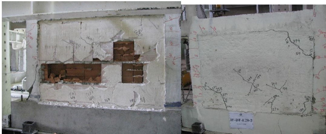
Figure 2.8 Left: Early shear failure of specimen IF-SF-E20. Right: Specimen IF-DF-E20-2 at failure. (Sharbatdar and Tajari 2021)
