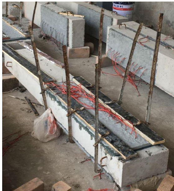
Figure 3.12 Installation of prefabricated strengthening layers. (Yang et al. 2020)
