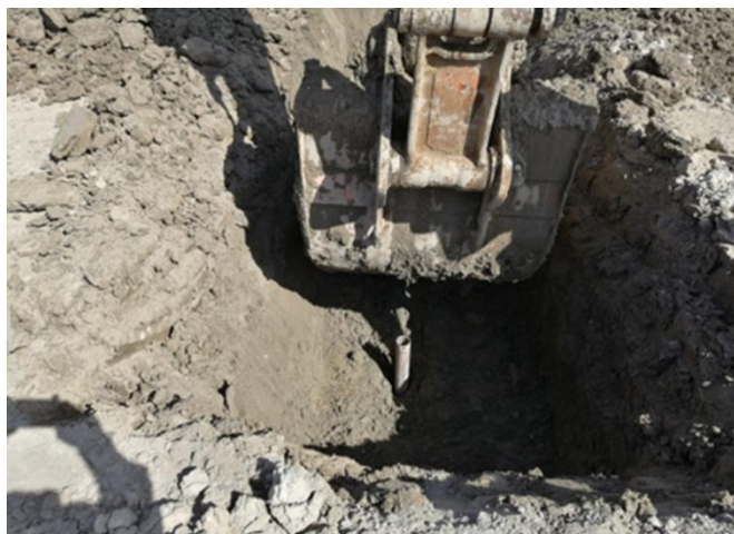
Figure (5) shulby sample for undisturbed soil
