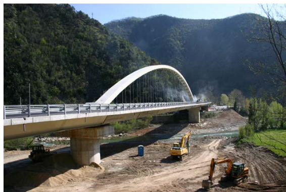
Figure 3: Deck of r.c. arch bridge
