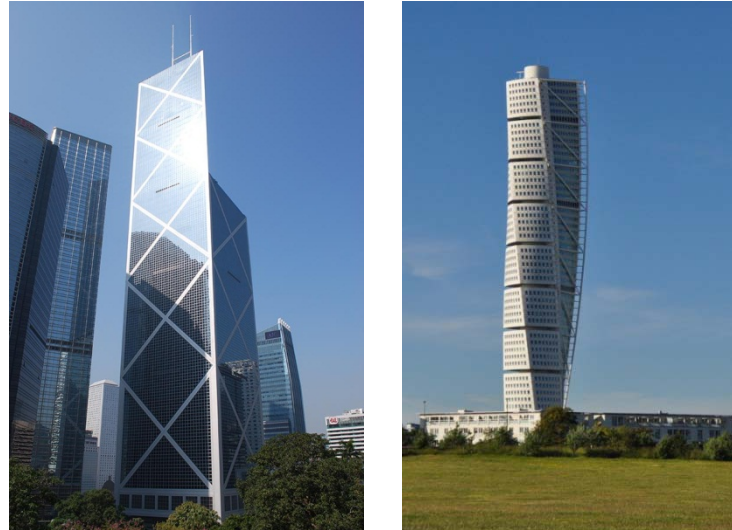
Figure 13: a) Bank of China, Hong Kong; b) Torso Tower, Malmo
