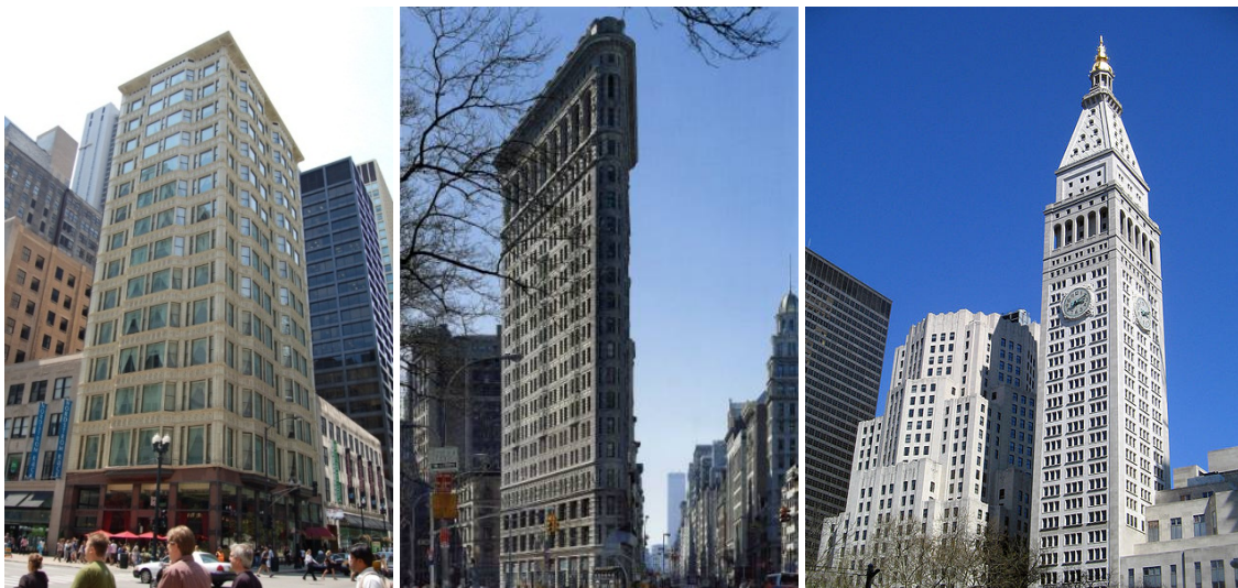
Figure 3: a) Reliance Building, Chicago; b) Flatiron Building, NY; c) Metropolitan Life Insurance Company Tower, NY
