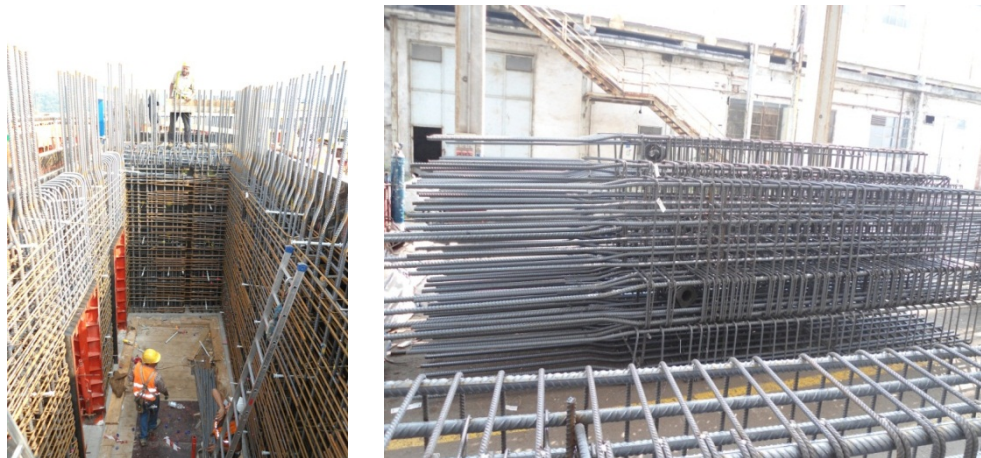
Figure 19: Self climbing scaffoldings and preassembled steelcages
