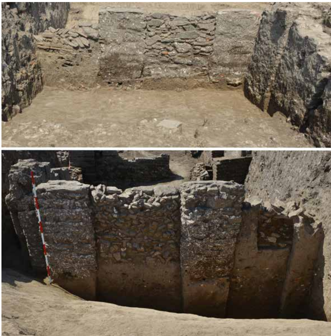
Fig. 4 Wall 2 (northern wall); upper- view from the south, lower-view from the north
