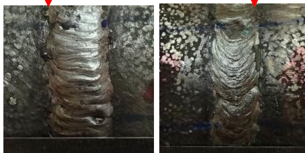
Figure 5. Location 1 (welded with Castolin 6825 electrode) and location 2 (welded with PIVA 25/20 B electrode) in pipes.
