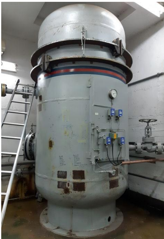
Figure 3. The pressure vessel 970 at RHEBB.
