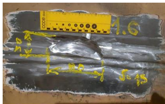
Figure 5. Welding groove after the removal of defect 1.6.
