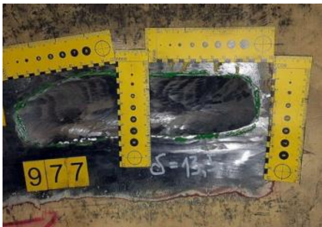
Figure 6. Welding groove after the removal of defect 2.5.
