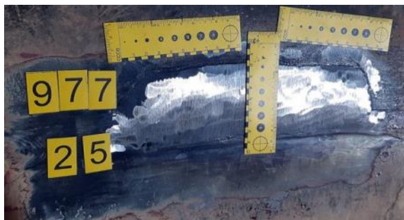
Figure 12. The inner surface after the repair - vessel 977.
