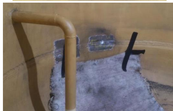
Figure 4. Working environment before repair welding.
