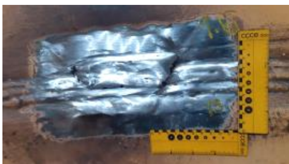
Figure 2. Position and size of defect 1.6 in vessel 977.
