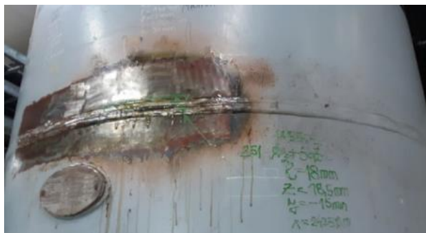
Figure 13. The outer surface after the repair - vessel 977.
