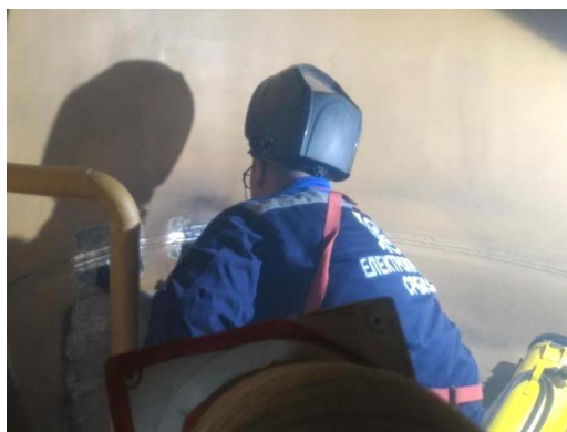
Figure 14. Interpass temperature measurement.
