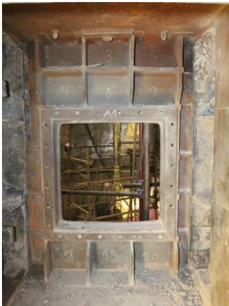
Figure 11. The reconstructed Kaplan turbine runner manhole welded structure.
