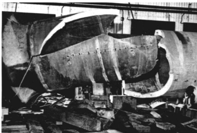
Figure 5. Large thick-wall pressure vessel – an ammonia converter, fractured because of a crack in HAZ. Slika 5. Velika posuda pod pritiskom – konvertor amonijaka, polomljen usled prsline u HAZ
