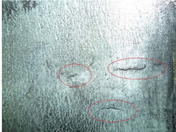
Figure 3. Crack detected by MT.
