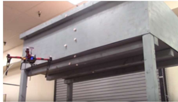
Figure 18: Hosing side of bridge deck
