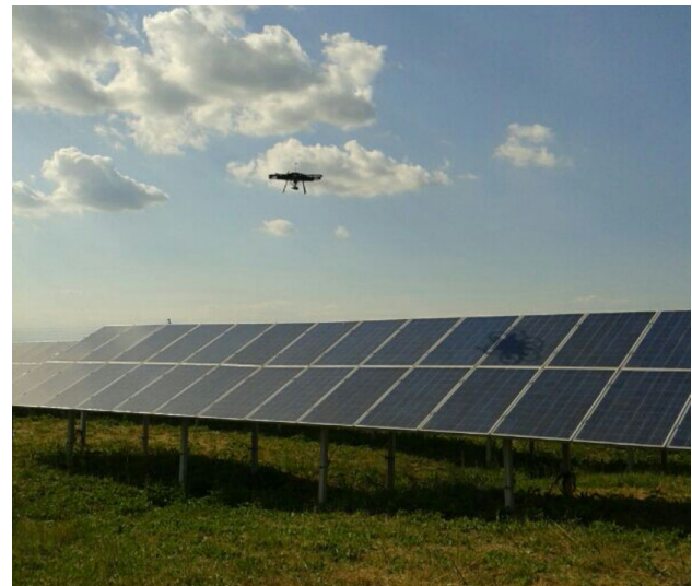
Fig. 6 PV modules inspection at PV plant in north of Italy by Nimbus PPL-610 UAV
