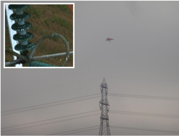
Fig. 1 Example of inspection process of transmission lines performed by Nimbus EosXi UAV in Italy
