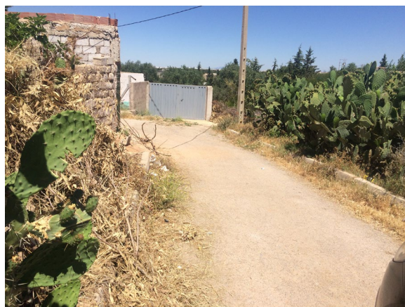
FIGURE 3. THE UNFINISHED ROAD IN THE DOUAR TLALSA, BLOCKING THE RESTRUCTURATION OPERATION LEAD BY THE COMMUNE
