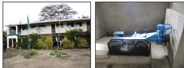
Fig. 1. Ngarenanyuki Secondary School (TZ) – Banki turbine generator.
