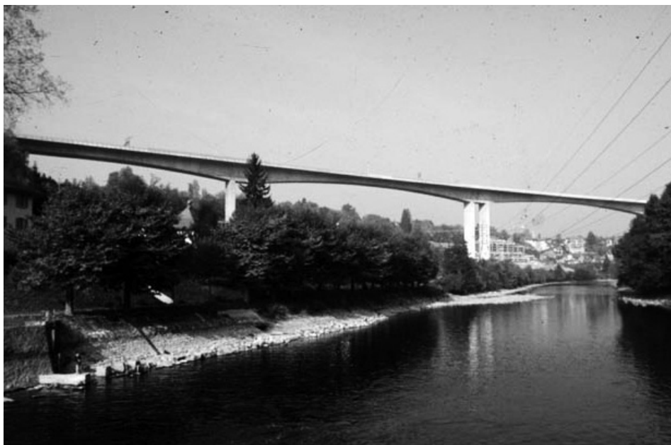
FIG. 7. PONTE A FELSENAU_MENN_1974 (WWW.CHRISTIAN-MENN.CH).
