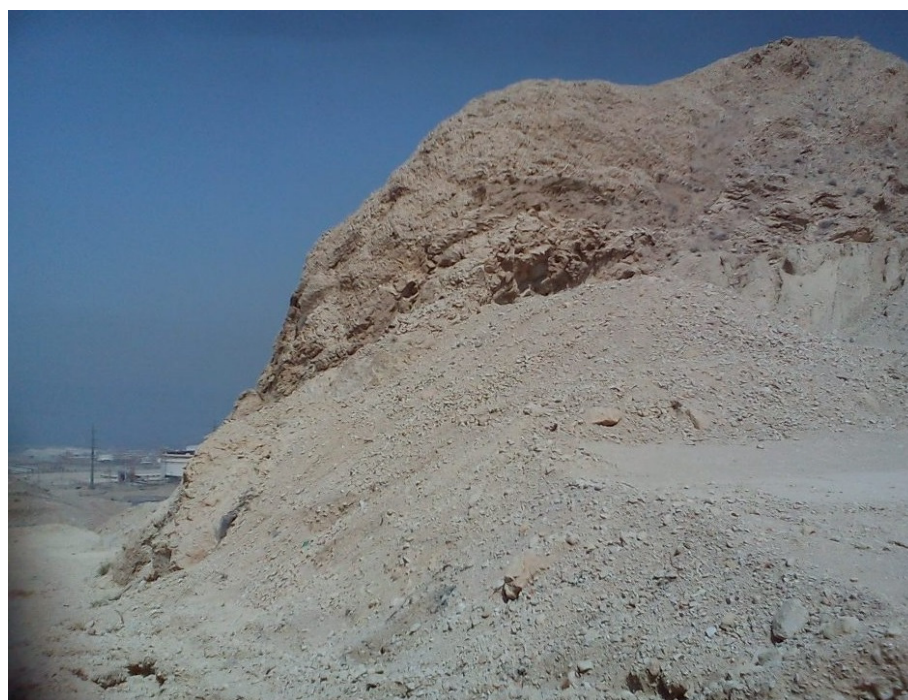
Figure 5. A view of the selected slope in the South Pars region.
