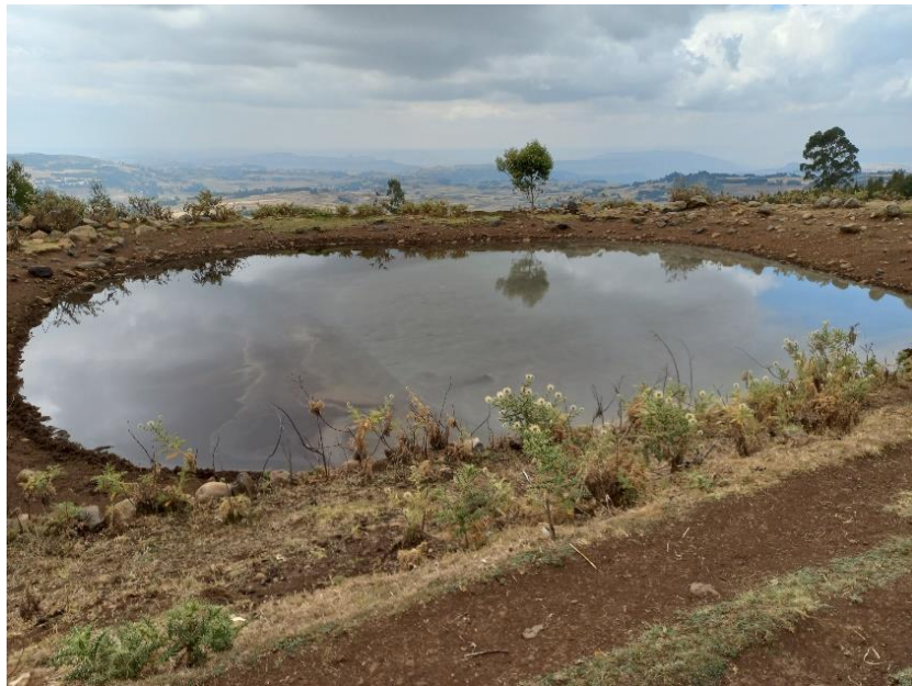
Harvested water mainly used for livestock drinking, the poor management has resulted with siltation problems
