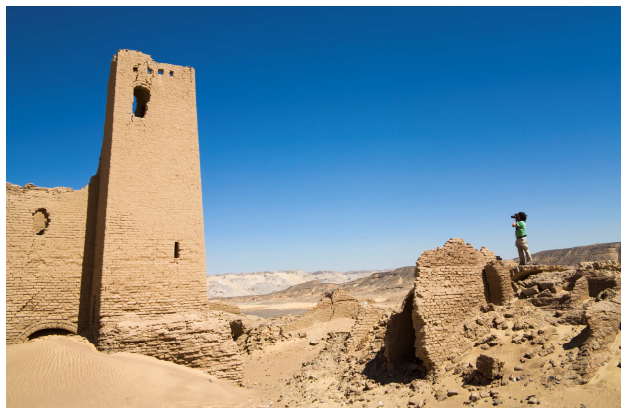
Figure 2. The photogrammetric survey of the castle tower.
