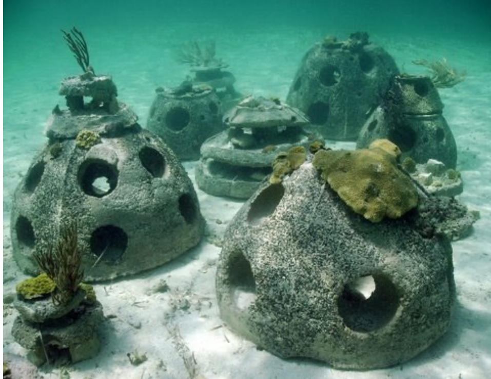
Figure 3 . Pictured here (front) are reef balls installed in a tropical setting for the purpose of coral reef restoration. The reef balls in this image are of similar size (3 feet) to the ones installed at the Dobbins Hill reef. Source ( http://www.reefball.com/brochure.htm )
