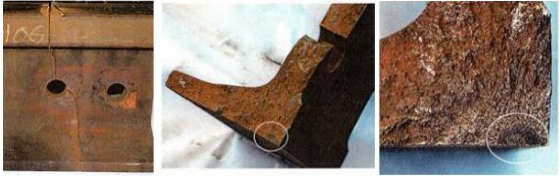
Figure 17. Showing a transverse fracture from corrosion pit defect [158].
