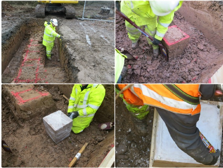
Figure 2-3 Sampling procedures for retrieving intact Cowden till block samples (Ushev, 2018)
