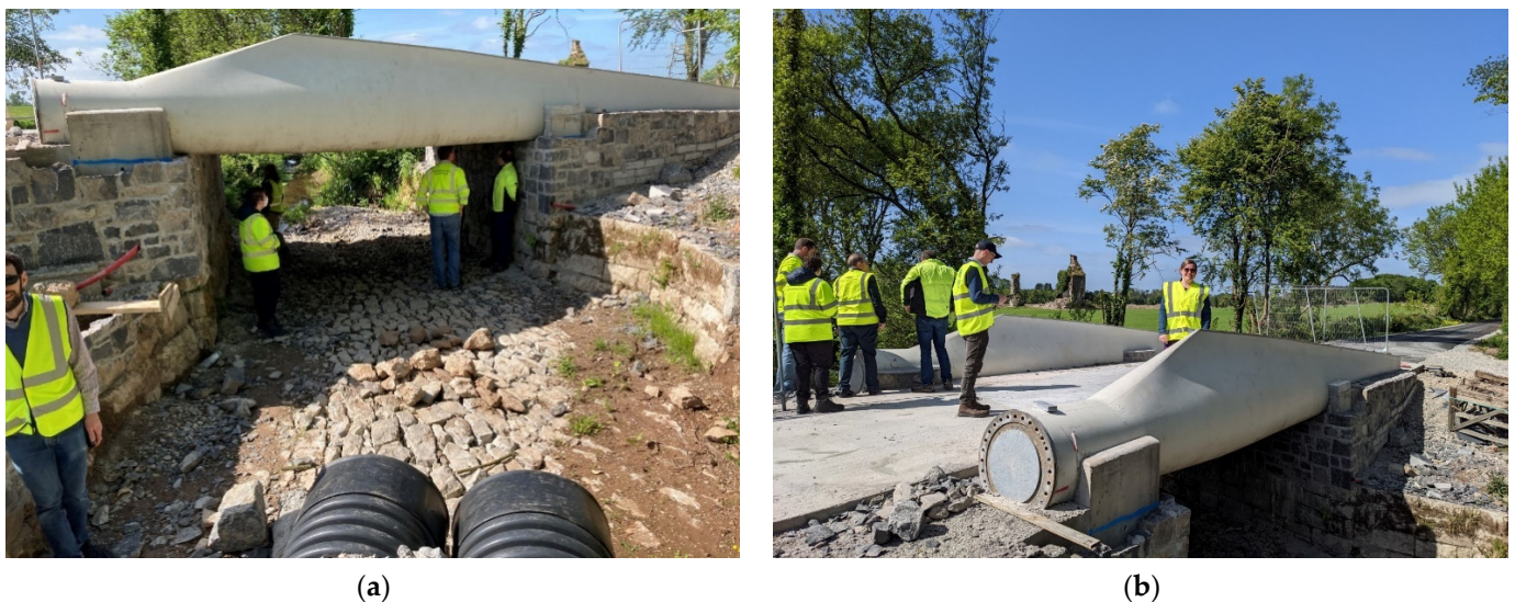
Figure 4. Re-Wind Network's first footbridge in Cork, Ireland, constructed from decommissioned wind turbine blades in January 2022: (a) Front view of the blade bridge; (b) Side view of the footbridge, Photo Credit: Re-Wind Network [104].
