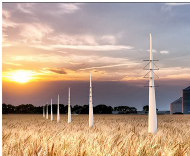
Figure 5. Rendered Wind turbine blade utility transmission poles to be constructed in Kansas, USA [93], Photo credit: Re-Wind Network [104].
