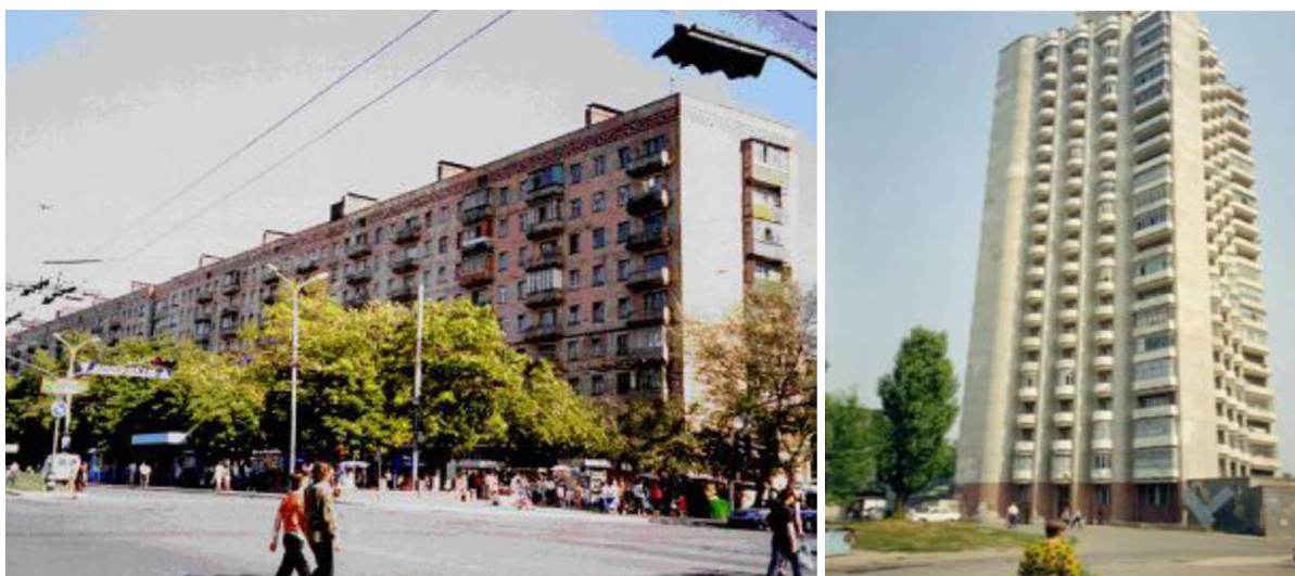
Figure 2.11 - The first low and high rise residential constructions OPC-free manufactured using alkali-activated cement concrete in the 1970s, Ukraine [54].
