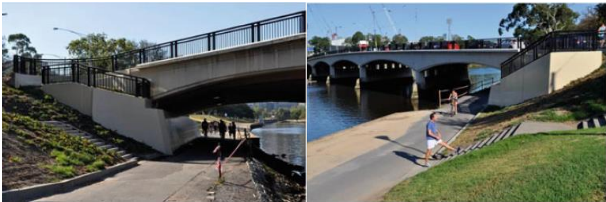
Figure 2.2 - E-Crete retaining wall at the Swan Street bridge in Melbourne, Australia [121].
