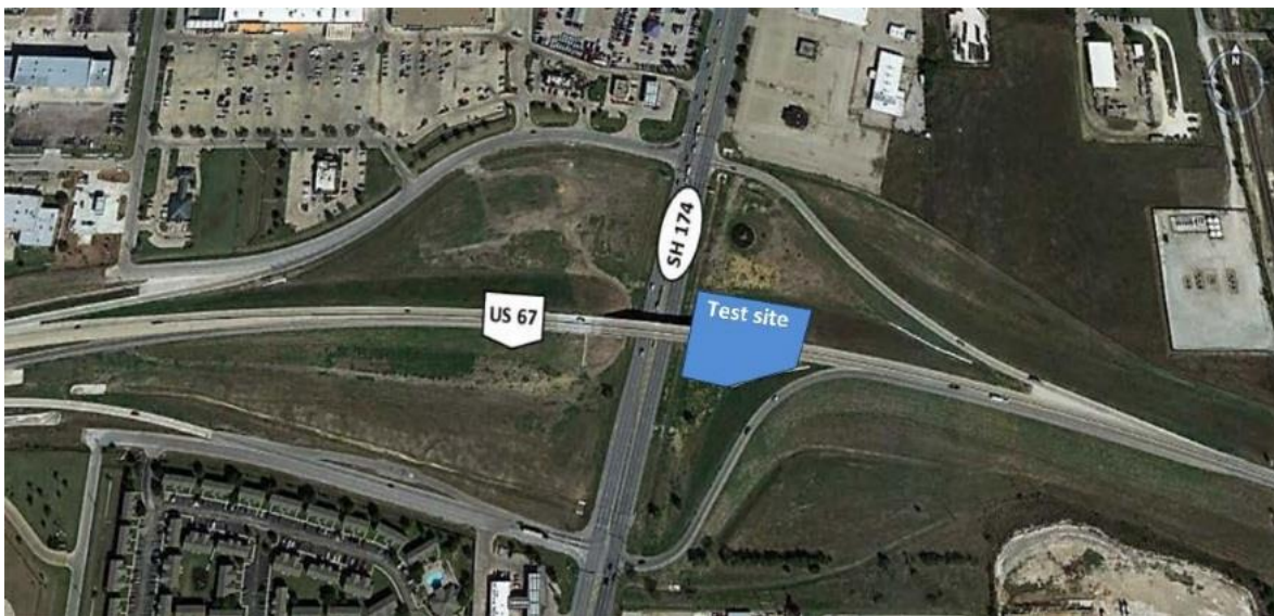
Figure 9. US 67 Bridge Approach Embankment Test Site
