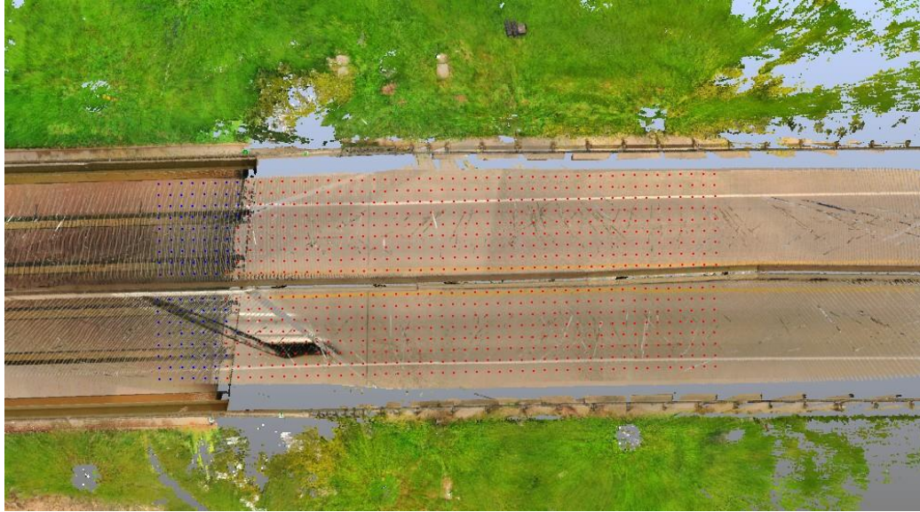
Figure 12. Set of Monitoring Points Placed over the Bridge Approach and the Deck
