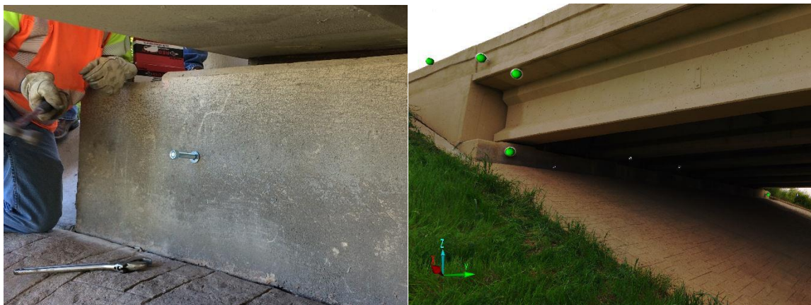
Figure 11. Installed anchors and reference spheres
