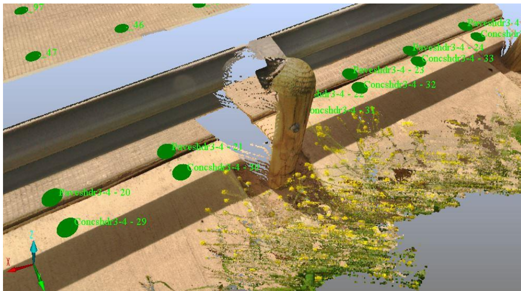
Figure 13. Monitoring Points on the Side Slope and Pavement Shoulder
