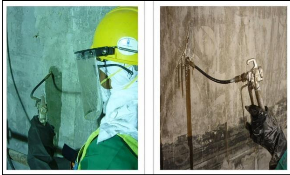
Figure 9.9. Injection of Epoxy Resin into the Holes (54).
