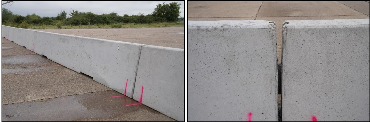
Figure 5.2. Single-Slope Barrier prior to Test No. 440590-01-B1.
