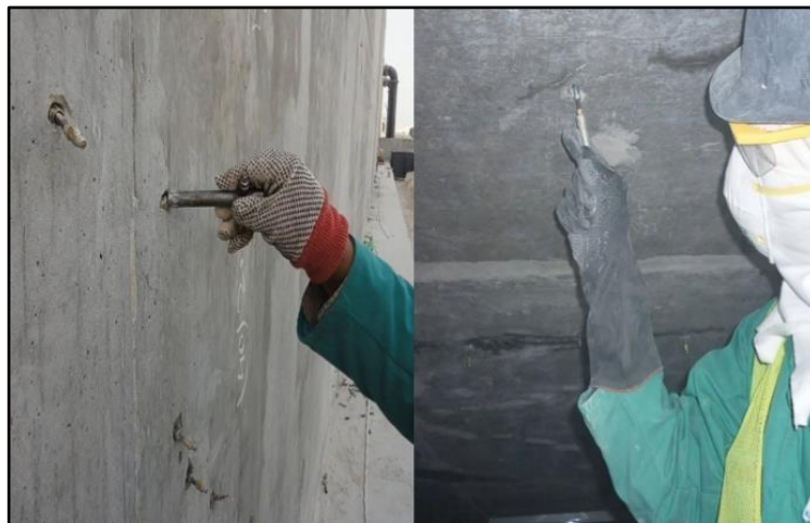
Figure 9.8. Installing Injection Ports (54).
