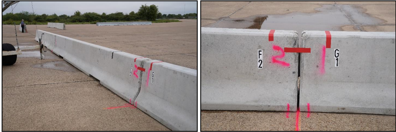
Figure 5.34. F-Shape Barrier prior to Test No. 440591-01-B4.
