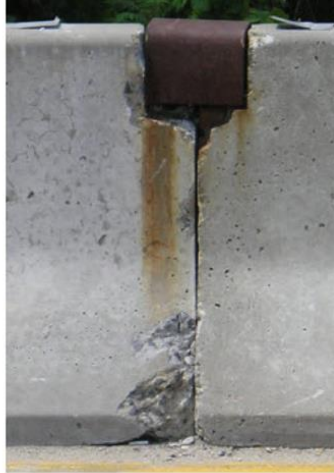
Figure 2.14. Corner Damage—NYSDOT (27).
