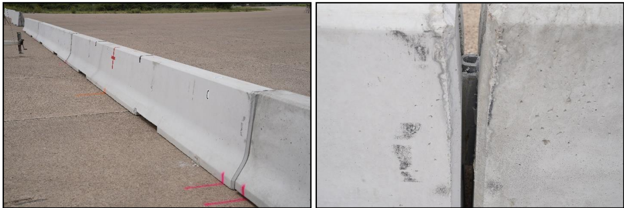
Figure 5.26. F-Shape Barrier prior to Test No. 440590-01-B3.
