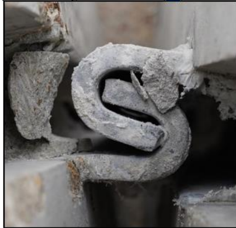
Figure 2.11. JJ Hook Connections: Top View of a JJ Hook Connection between Barrier Units.
