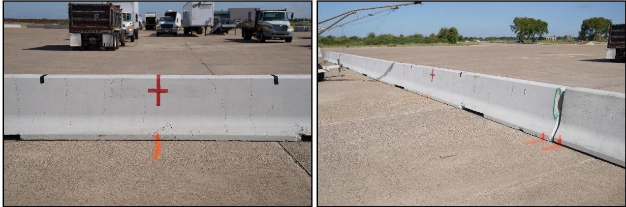
Figure 5.30. F-Shape Barrier prior to Test No. 440590-01-B11.
