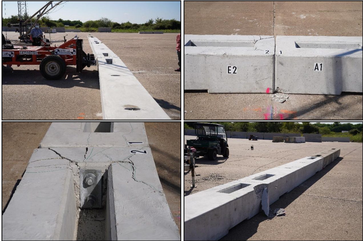
Figure 6.7. Low-Profile Barrier after Test No. 440591-01-B6.
