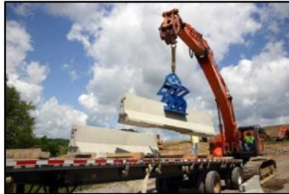
b. Single-point lifting (13)
