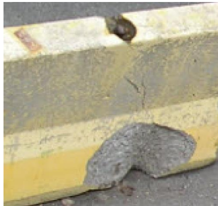
Figure 2.16. Unacceptable Barrier Due to Snag Risk—NYSDOT (27).
