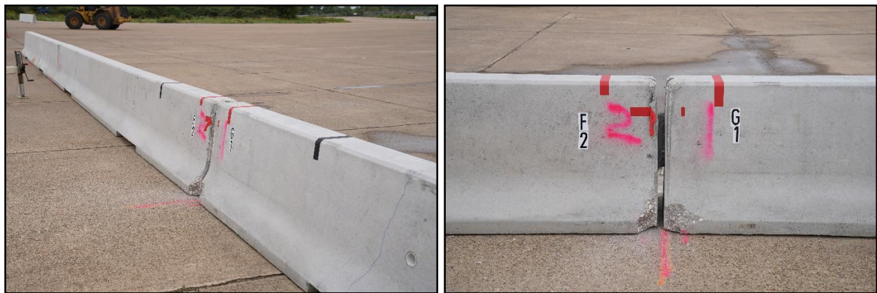
Figure 5.38. F-Shape Barrier prior to Test No. 440591-01-B12.
