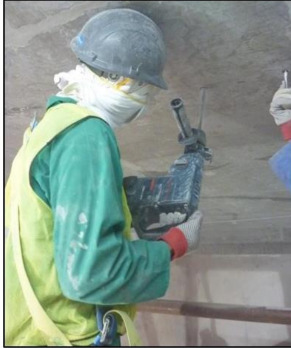
Figure 9.6. Drilling Holes in the Concrete Member (54).
