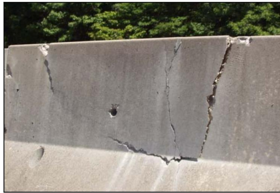
Figure 3.2. Unacceptable Barrier—IDOT (34).
