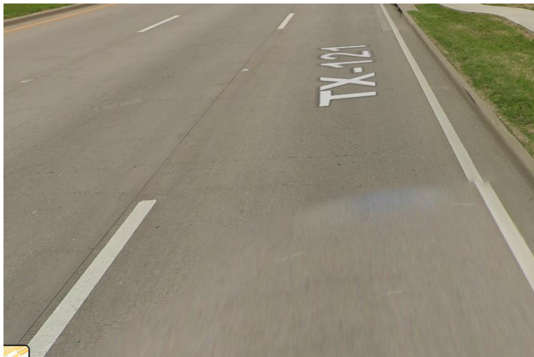
Figure A15. Presence of Curb.
