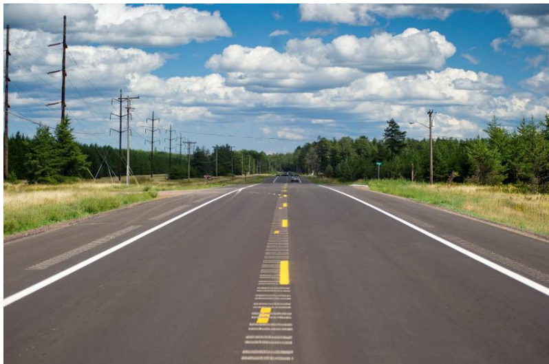
Figure A2. Centerline Rumble Strip.
