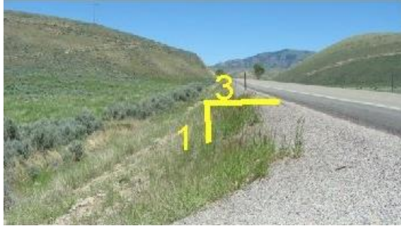
Figure A6. Example of Sideslope 1:3.
