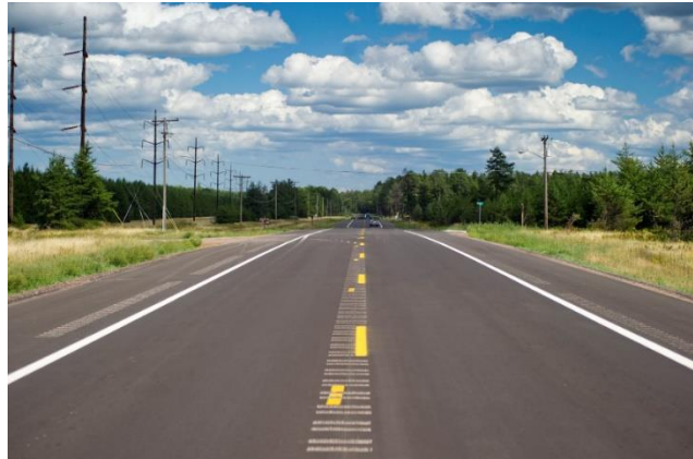
Figure A14. Centerline Rumble Strip.
