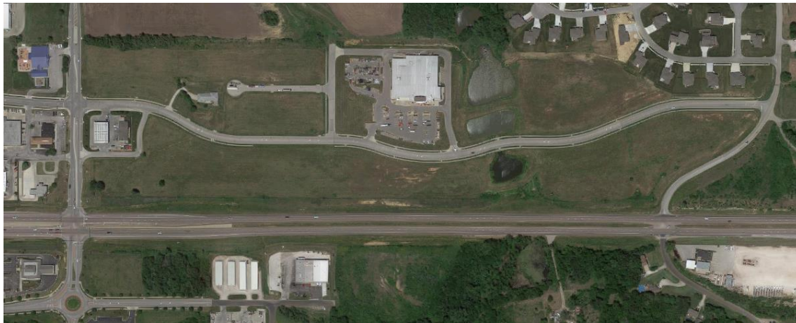
Figure 8: Service road funded by access management set-aside funds.
