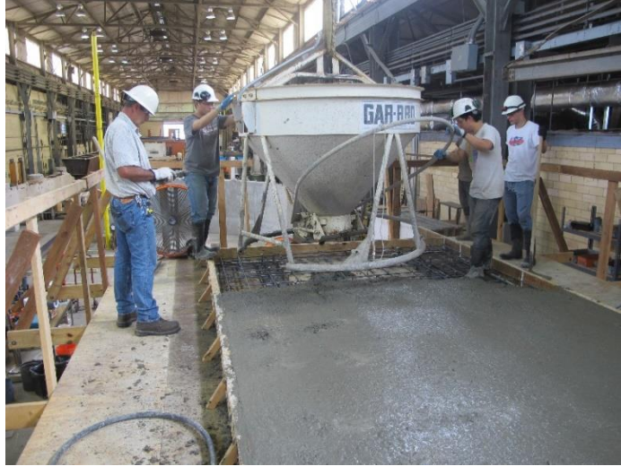
Figure 5-11 - Concrete Deck Casting - Tub #1
