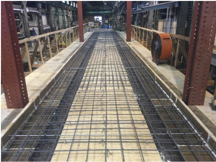
Figure 5-10 - Steel Reinforcement of Concrete Deck – Tub #1
