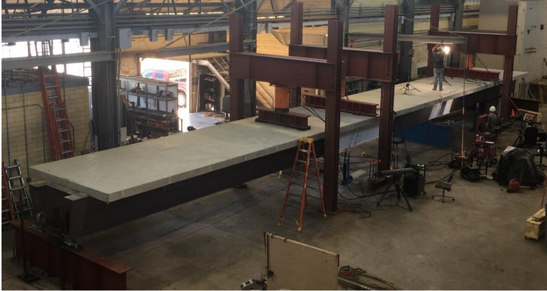
Figure 5-19 - Continuous Girder Test Setup - Tub #2
