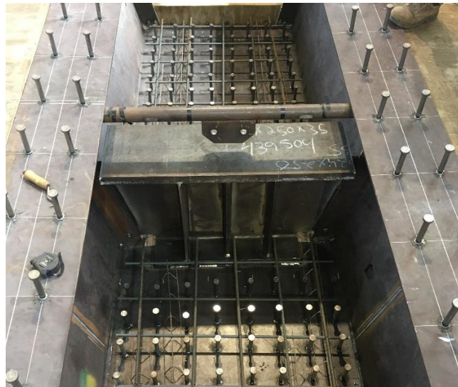
Figure 5-7 - Solid Diaphragm and Bottom Flange Reinforcement (before Casting) - Tub #2
