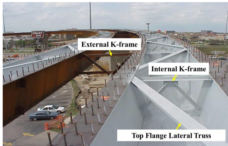
Figure 1-2 Typical Twin Tub Girder System during Construction
